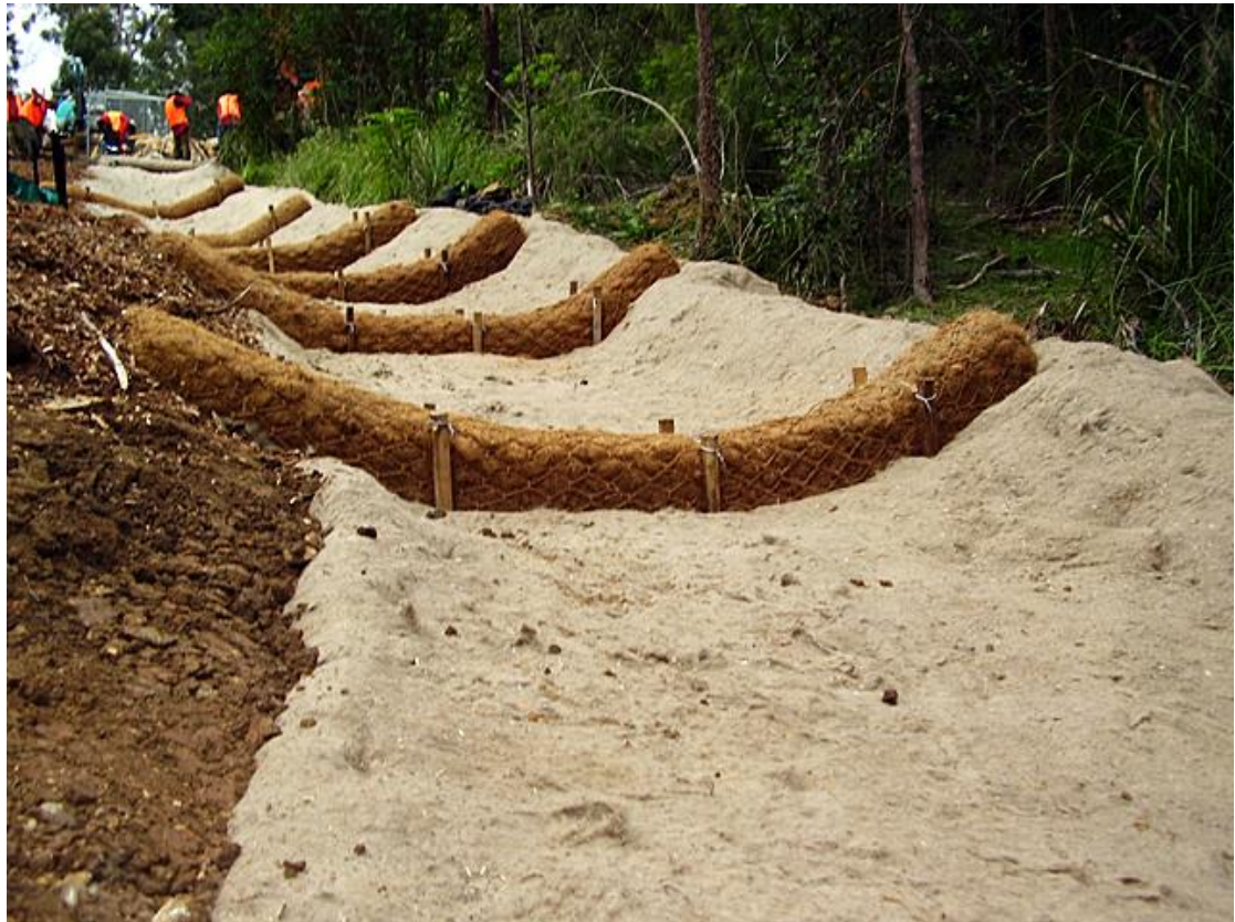
Figure 7: Typical Application of coirlogs and erosion control blankets
